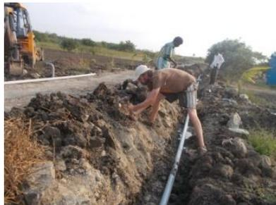
A very practical but critical achievement: we installed a pipeline for the irrigation of our plants. The purpose of the pipeline is to efficiently deliver water from the new well to the cultivation areas. It will help to reduce erosion, conserve water, and protect the water quality. This will be
